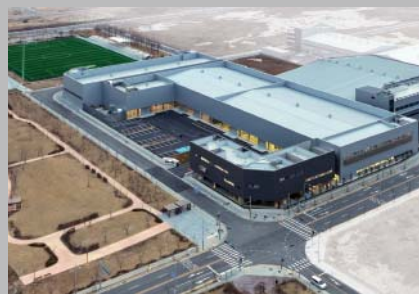
Factory in Sihwa MTV Complex
